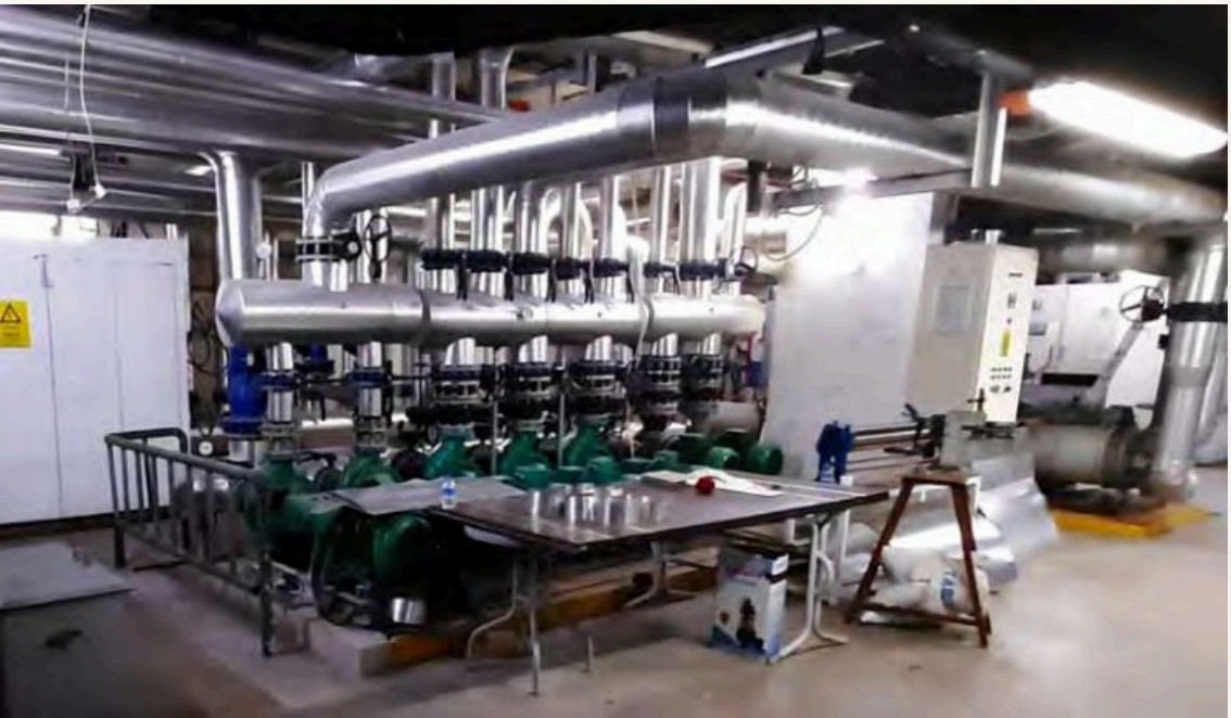
Boiler Room Thermal Insulation
